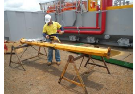
Drilling rig Site measure
