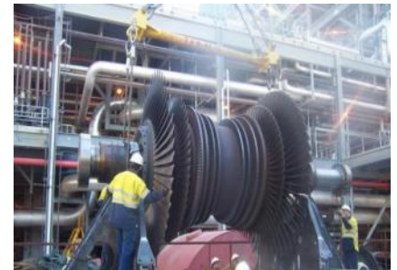
Millmerran Power Station, QLD Turbine Transport Frames Design, Drafting, Certification
